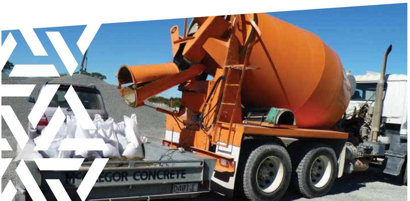
Below: The set up at McGregor's Concrete in Winton for filling sand bags March 2015
