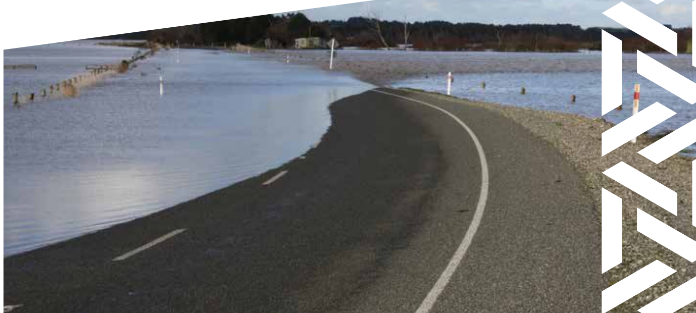
Significant flooding across the road from the Mataura River at Titiroa
